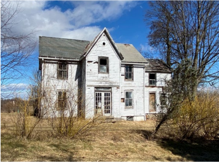
Fig. 23. Birdsall House, 300-304 Willow Tree Rd. The projecting entrance bay with its Gothic Revival gable was grafted on a traditional center-passage-plan house.
